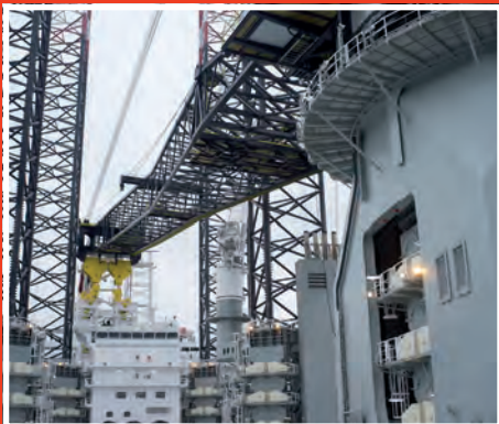
▲ View from the aft towards the accommodation, with the main crane resting on monkey island.
