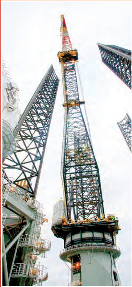
▲ Auxiliary crane, three of the six support legs and the main crane.
